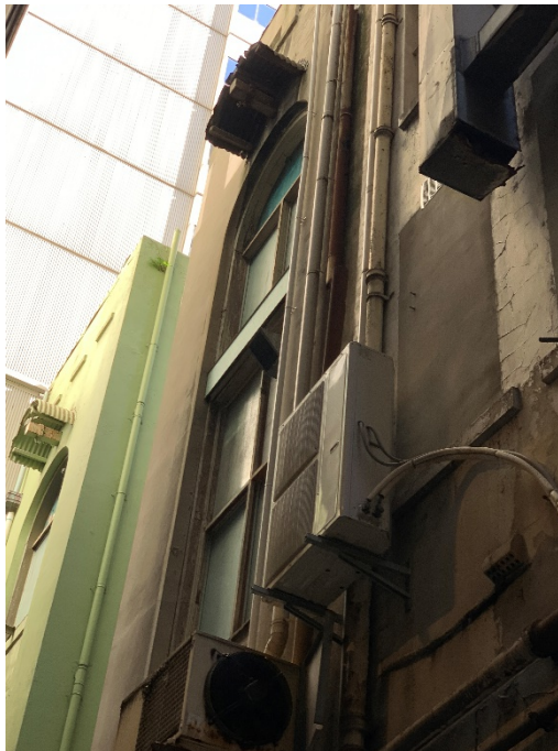
21 Detail view of rear of 15-17 Hunter Street showing arched openings, corrugated iron hoods over hoist and window detailing
